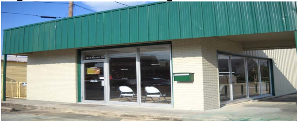
The clinic at 1013 Barrow Street is ready for business.
